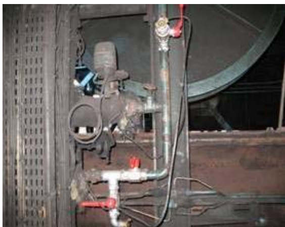
Fig. A6.1 System of air by-pass in Carling
