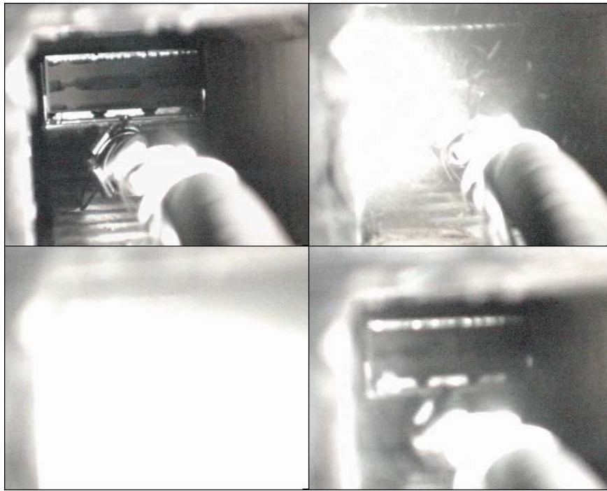
Fig. A6.25 Photos of regenerator brickwork inspection with the Prototype 2 inspection/cleaning system with simultaneous operation of the cleaning equipment left top before start of cleaning right top start of cleaning left bottom during cleaning right bottom after cleaning
