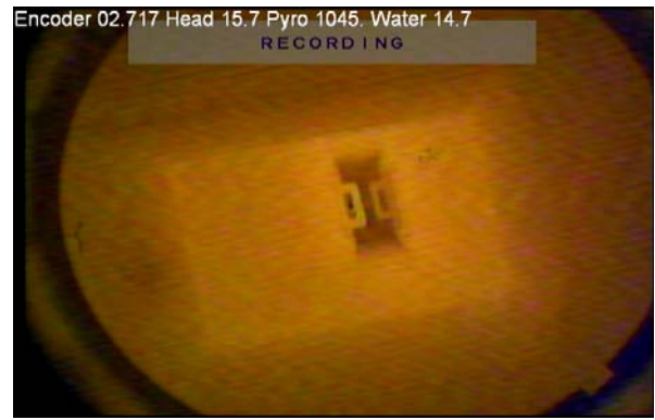
(b) 2.7 m from battery top showing 2 burners
