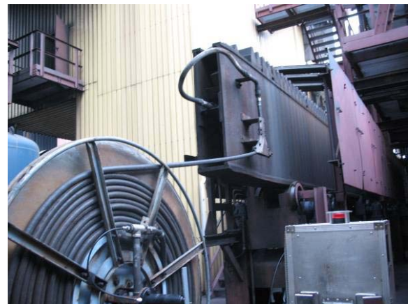
Fig. A6.8 Coaxial cable in the decarbonising air pipe in Dillingen
