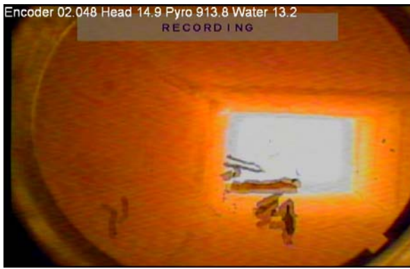
(a) 2 m from battery top showing deposits in flue
