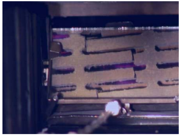
damaged brickwork – cracks
