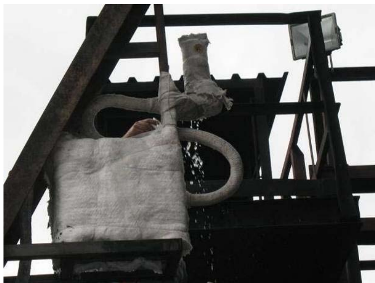
Fig. 11 Insulated camera, electronics and cables
