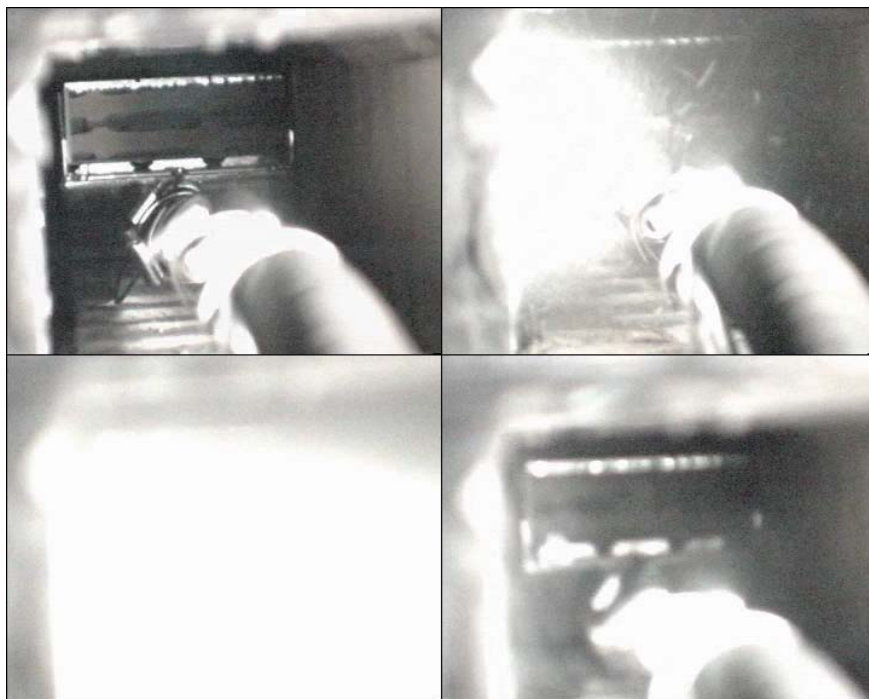
Fig. 37 Photographs of regenerator brickwork inspection with the Prototype 2 inspection/cleaning system top left before start of cleaning top right start of cleaning bottom left during operation of cleaning equipment bottom right after operation of cleaning equipment
