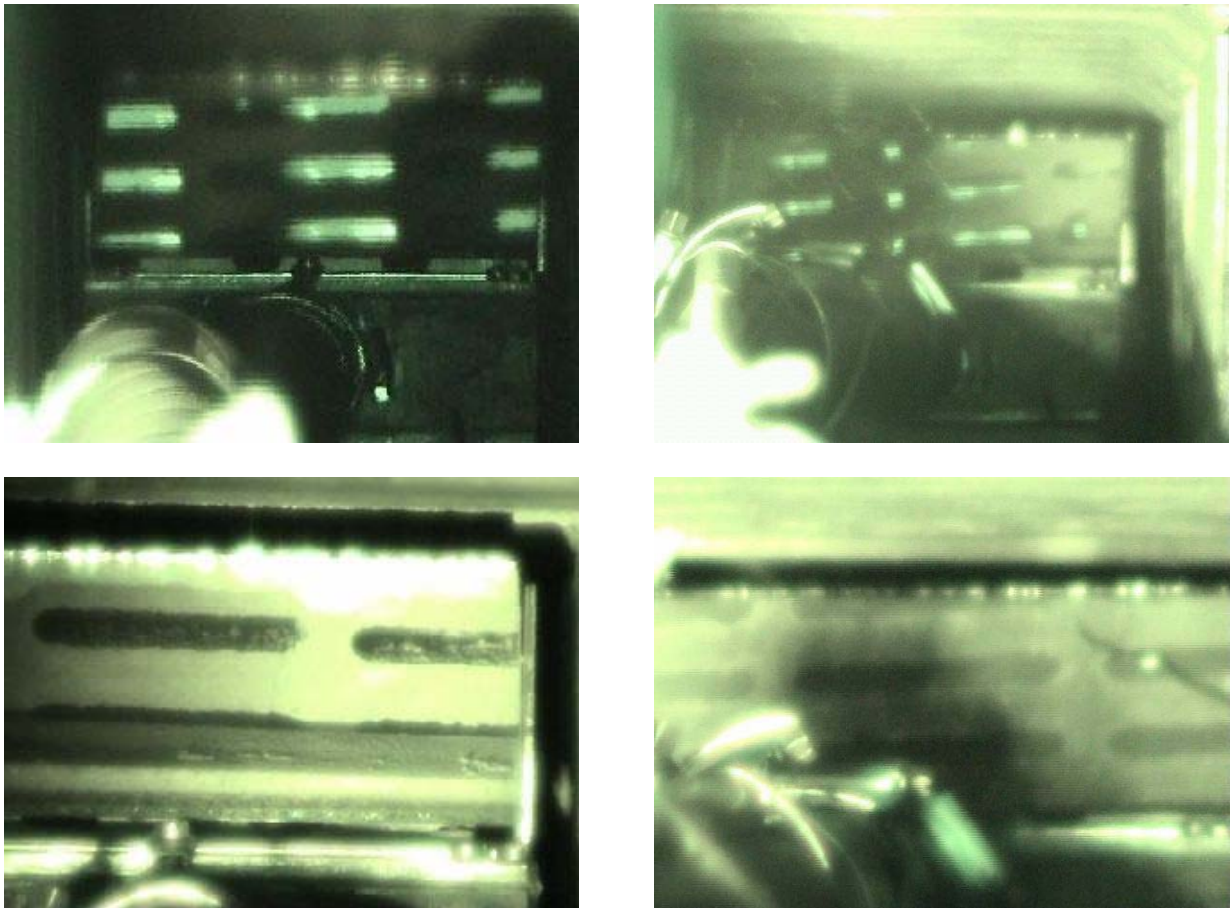
Fig. A6.24 Photographs of regenerator brickwork inspection with the Prototype 2 inspection/cleaning system without operation of the cleaning equipment (camcorder: IR-mode)
