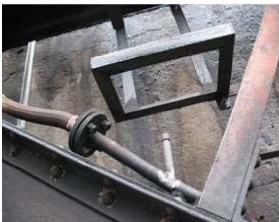
Fig. A6.3 Escape air pipe in Carling
