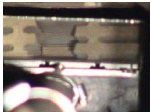
Fig. A6.23 Photographs of regenerator brickwork inspection with the Prototype 2 inspection/cleaning system without operation of the cleaning equipment (camcorder: visual mode)
