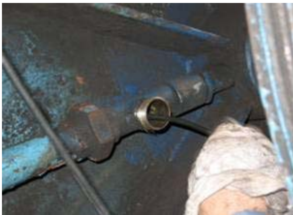
Fig. A6.7 Coaxial cable installation in Carling
