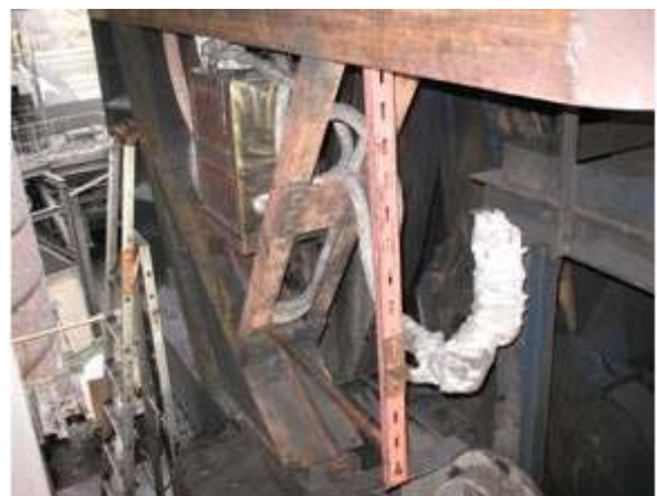
Fig. A6.10 Insulated camera head installed on the Carling pusher ram
