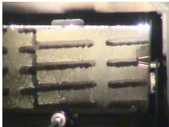
damaged brickwork – structural surface damages
